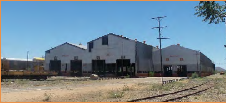
Figure 2 The Main workshops of SBC at Benjamin Hill, Sonora in 2017. Shortly after this photo was taken the shops were completely dismantled
